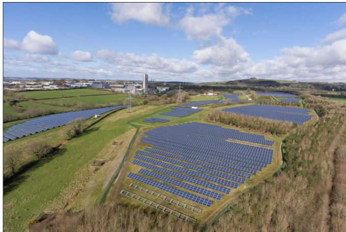
Solar panels that may yet help Langage produce green hydrogen
