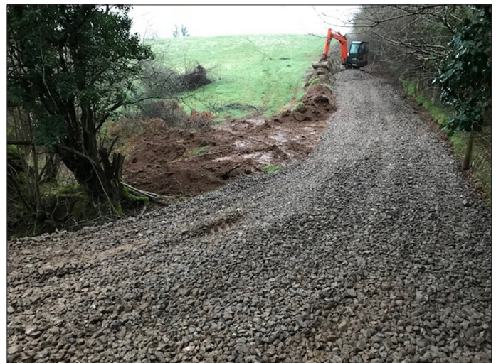
The track being excavated immediately next to the hedgerow
