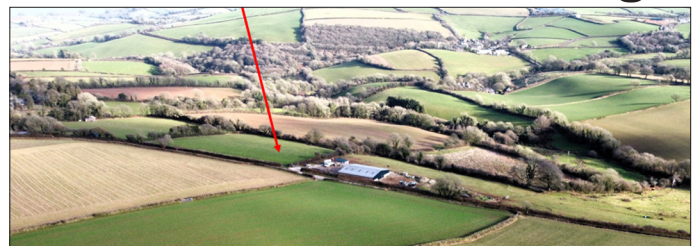
The existing building can be seen to the right
