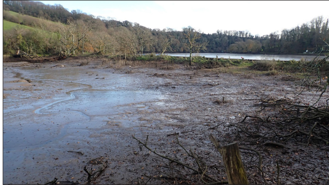
The Fleet Mill seawall as seen from the Marsh
