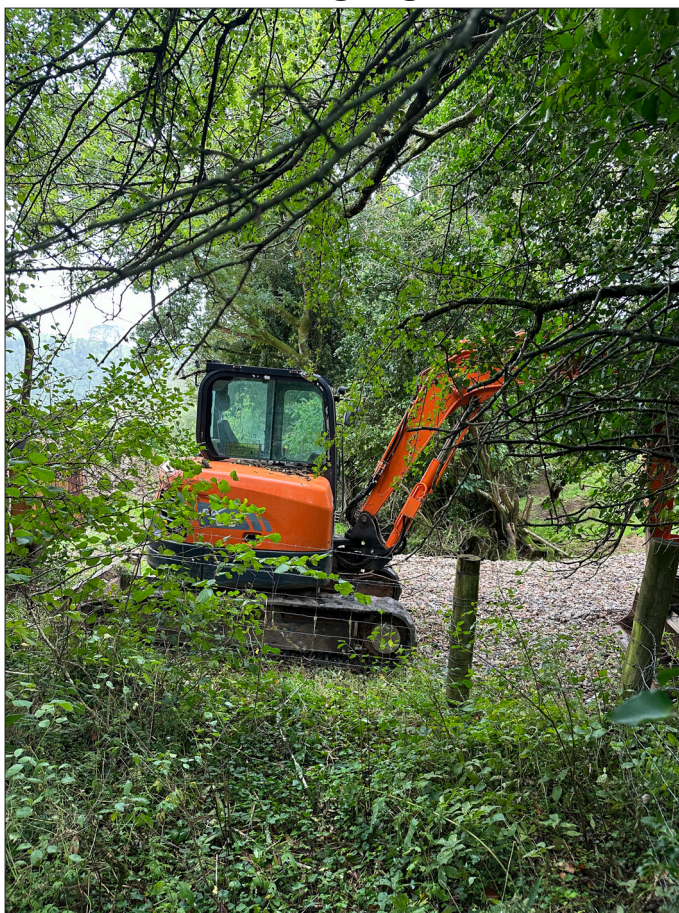
The digger on the track through the trees
